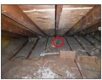
**2.5 Attic Insulation**: The attic floor insulation depth averaged approximately 8 to 10 inches. A more ideal depth for this type of insulation would be about 14-16 inches. As an improvement, you may consider additional insulation in the attic to help with energy conservation, lower humidity levels in the attic, and improved general comfort in the home.
