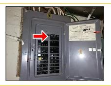
**8.4 Service Panel Wiring:** There is a "double-tapped" circuit in the electric panel. This is a condition where more than one hot wire is connected to a circuit breaker designed for only one wire. This should be corrected by a qualified electrician.
