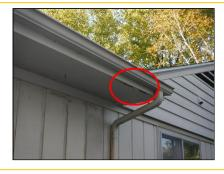
**4.4 Exterior Wall Penetrations:** Exterior wall penetration had gaps that should be sealed to prevent moisture and pest intrusion.
