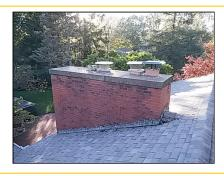
**1.4** Chimney at Roof: There are a few cracks in the concrete chimney crown that have had sealant applied in the past and will require re-application of sealant in the future as a maintenance item to prevent water intrusion which can damage the brick.
