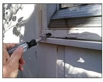
4.3 Eaves, Soffit, Fascia: There is some damage to the fascia trim at the South side of the Garage that may be related to past Wood Destroying Organism (WDO) activity. The inspector did not observe any active signs of insects. Repair of the fascia trim will be necessary to prevent damage from moisture intrusion.
