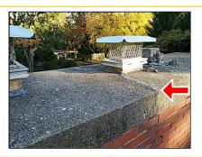
1.4 Chimney at Roof: It appears that one of the abandoned chimney flues was plugged at some point in the past and now the weatherproofing of the plug has deteriorated. This should be sealed against water intrusion by a qualified masonry contractor. This flue was likely used to vent an older furnace.
