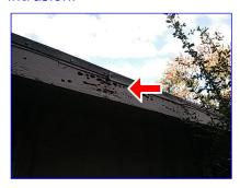
**8 Eaves, Soffit, Fascia:** There is a loose area of soffit at the West side of the home that requires additional securing to help prevent pest intrusion.
