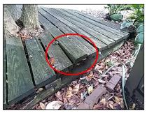
**3.5 Deck:** The Inspector recommends treating the deck with a stain/sealer to increase the longevity of the decking material and to reduce the likelihood of slipping.
