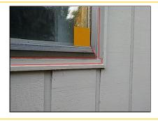
**4.1 Window Exteriors:** The wood frames at the Basement windows require priming, caulking, and painting to protect the condition of the wood.
