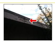
**4.3 Eaves, Soffit, Fascia:** There is a loose area of soffit at the West side of the home that requires additional securing to help prevent pest intrusion.
