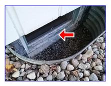
**Window Exteriors:** The window sills at the West side of the home are weathered and deteriorated and require repair.
